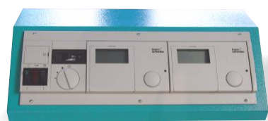
Boiler regulation Cm with built-in regulators E8.0634 i E8.1124
