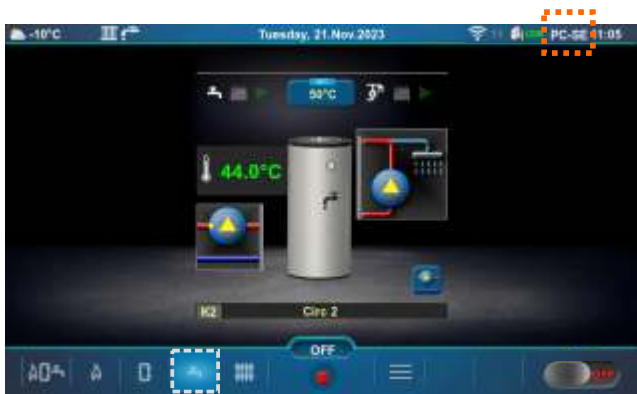
Domestic hot water (DHW) tank screen (PC-SE)
